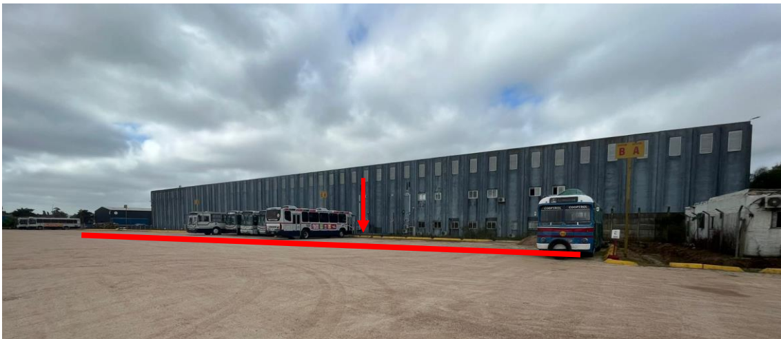
Veracierto Plant – area of chargers to be installed
