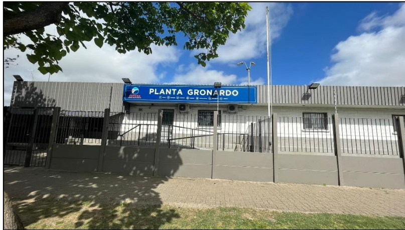
Photograph 13 Gronardo Plant and its surroundings
