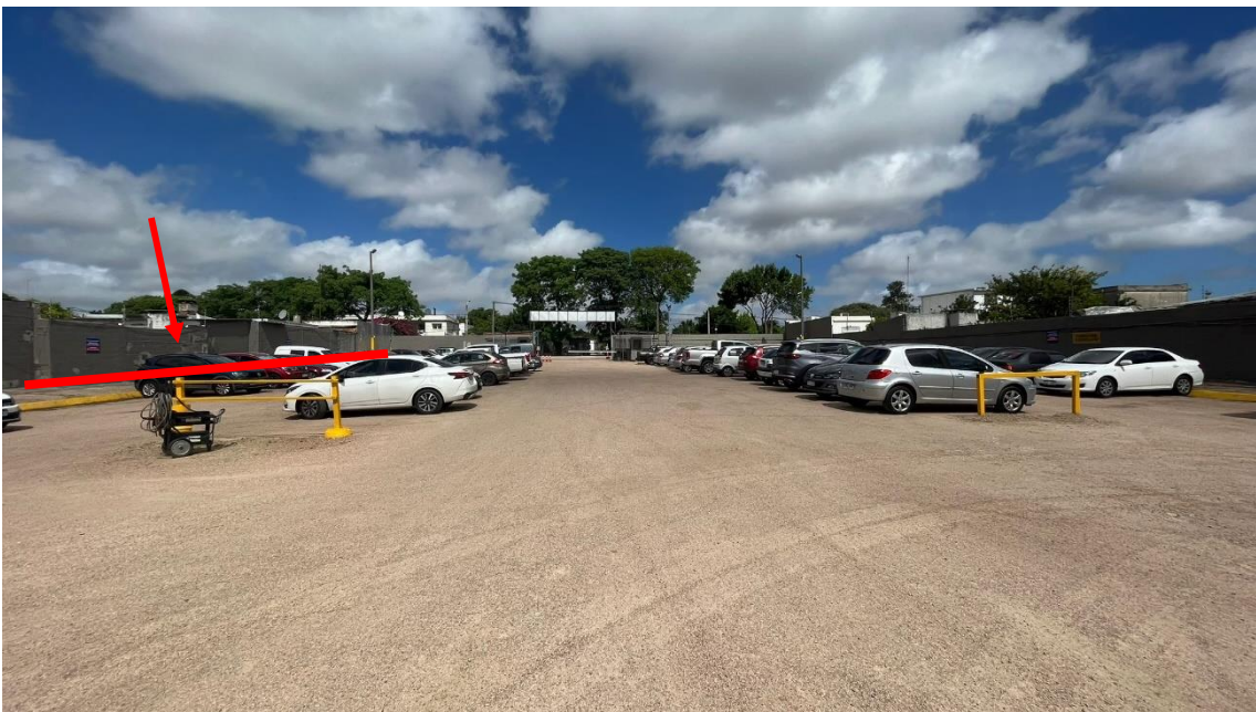
Canary Islands Plant – area of chargers to be installed
