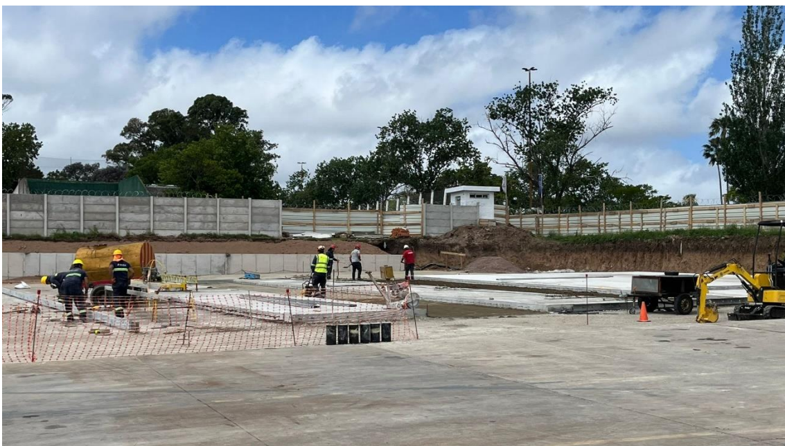
Añón Plant – charger area to be installed
