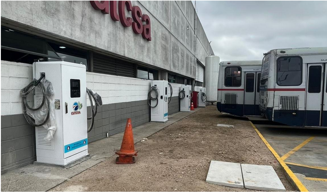
Juan A. Salgado Plant – already renovated loading area
